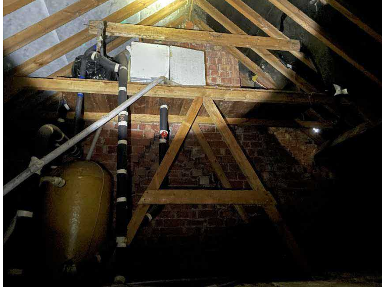
Plate 4 –House, internal roof void.
