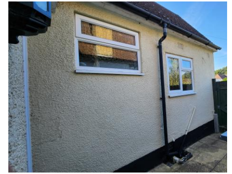
East side Elevation photo 2
