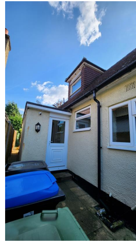
East side Elevation photo 1
