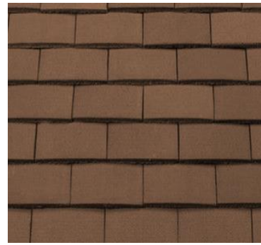
Tile cladding to existing
