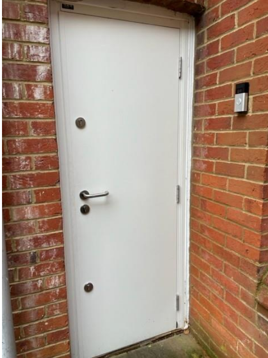
The steel door at The Cycle Co, Shawford
