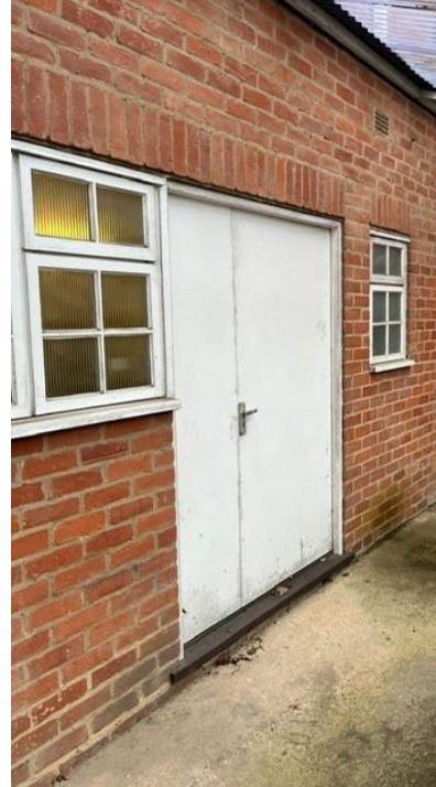
The existing back door at 86, The Hundred
