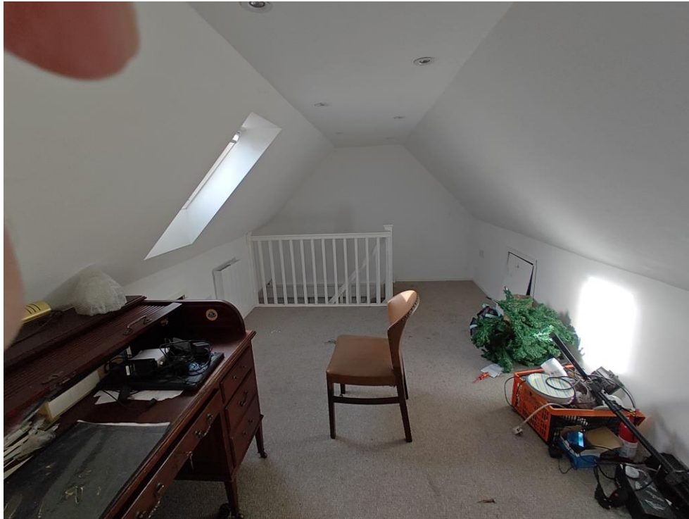
IMAGE 7 : looking to rear elevation showing stairs to first floor
