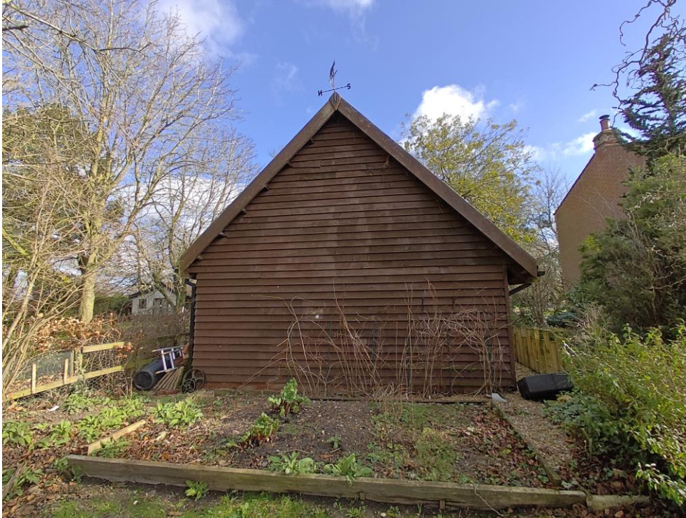
IMAGE 3 : rear elevation to private garden – NOTE 1 : trees seen are off-site
