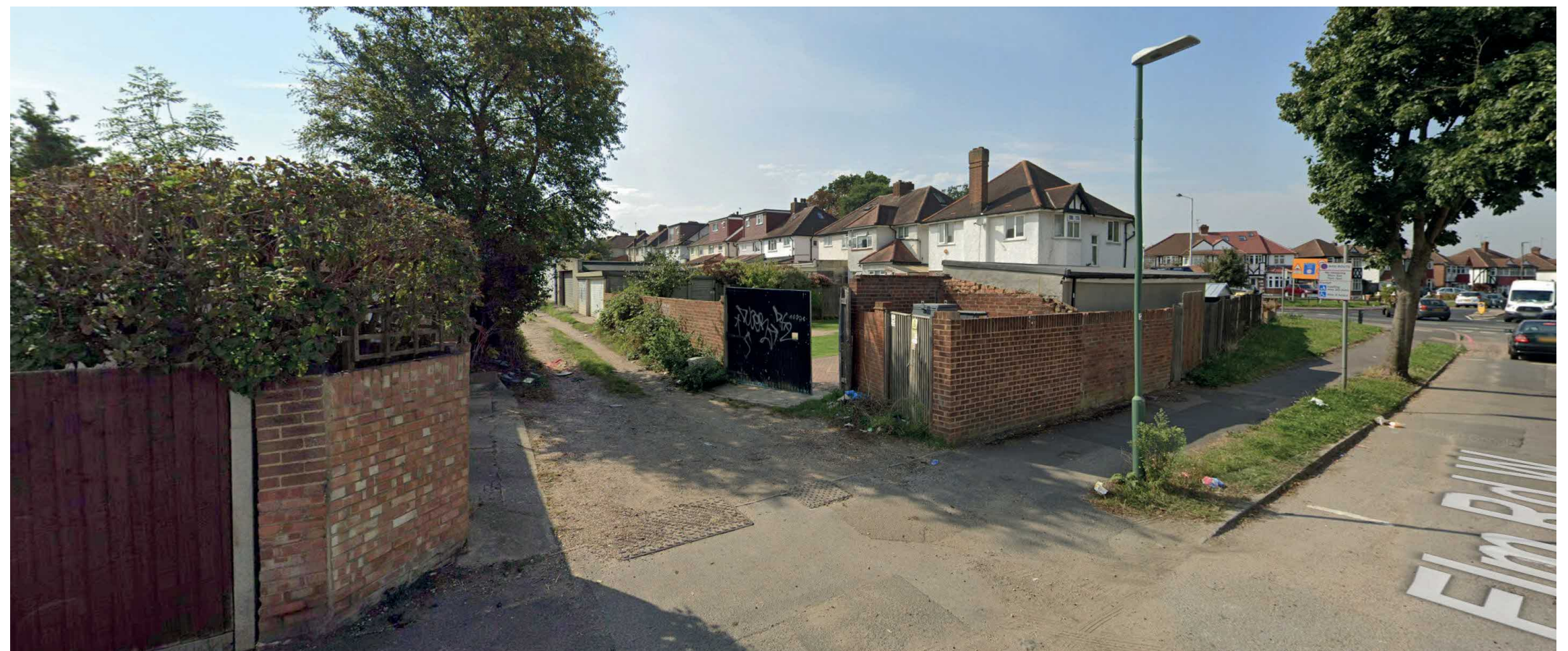
The rear of the site with the existing rear access and parking arrangements.
