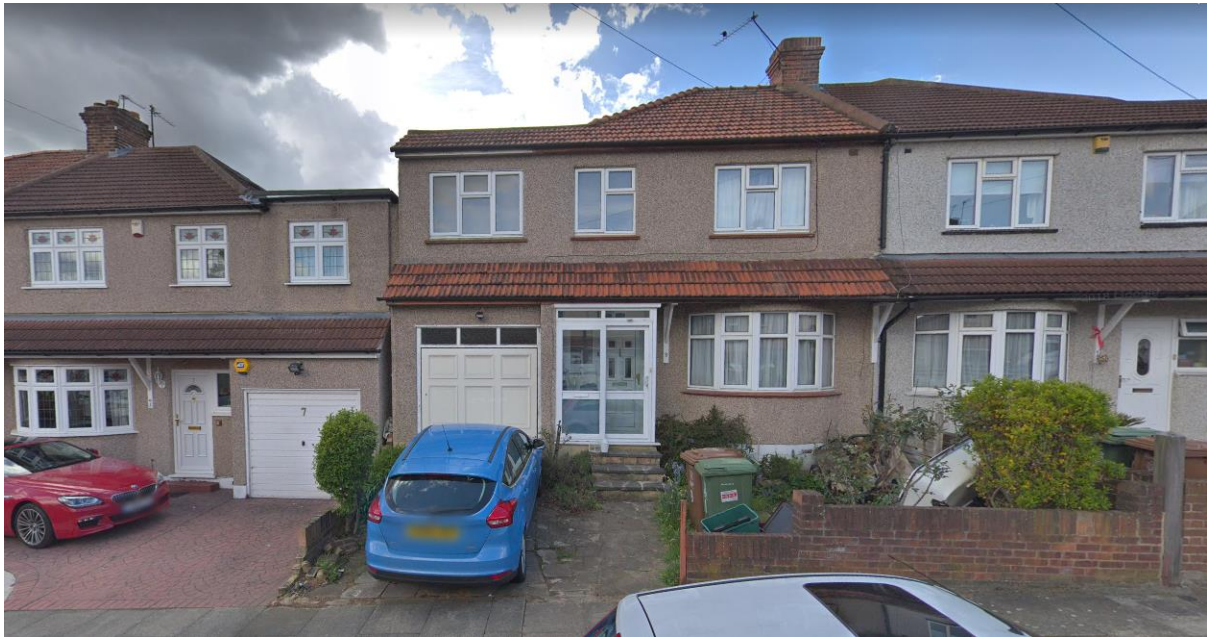
Photo of No 7 & 9 Martin Rise – Front wall is not set back with a room at front at first floor with flat roof
