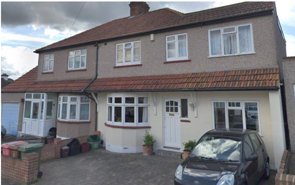
Photo of No 3 and 1 Martin Rise – Front wall is not set back with a room at first floor level.
