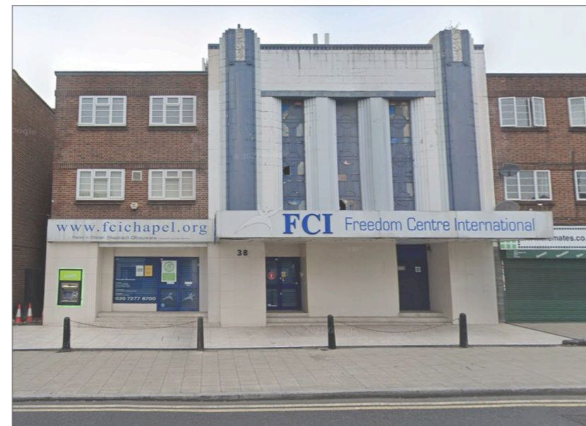
1 Freedom Centre, Locally Listed Upper Wickham Lane, Welling
