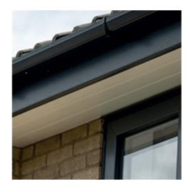
**4 - GUTTERS AND DOWNPIPES** 112mm UPVC Half Round Guttering & 82mm Dia. Downpipes. 7016 Grey
