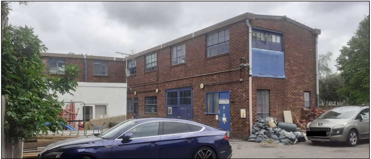
Figure 7: Existing buildings on site.
