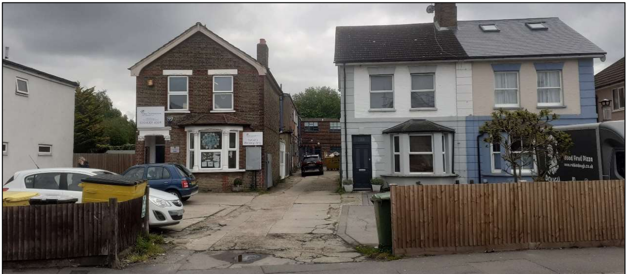
Figure 6: 41 Church Road and access to rear commercial units.
