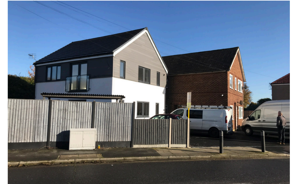
View showing the existing buildings at the site
