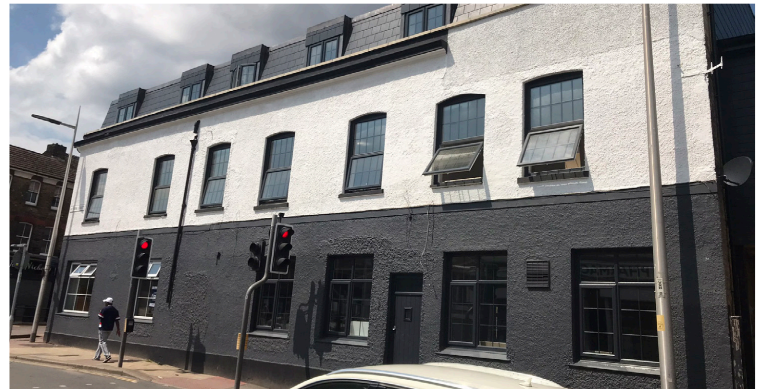
Completed scheme with additional storey, Gillingham
