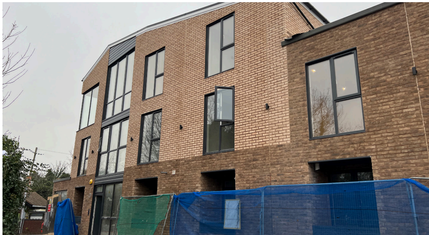
Completed micro-apartments scheme, Dartford
