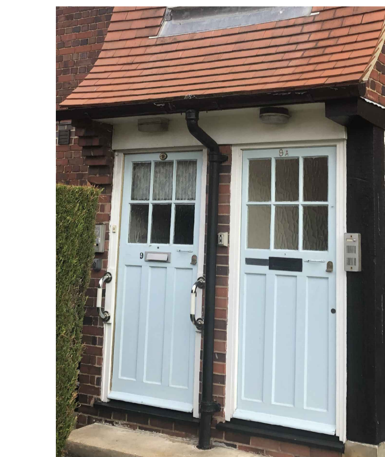
Existing Doors In-Situ NTS
