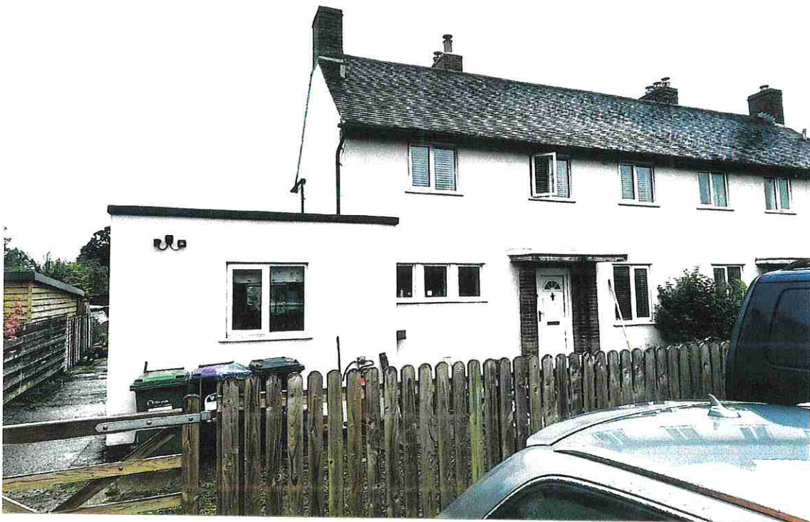
PHOTOGRAPH 1 - GENERAL VIEW OF THE ROADSIDE FRONTAGE OF No.10 RUSHBURY ROAD.
