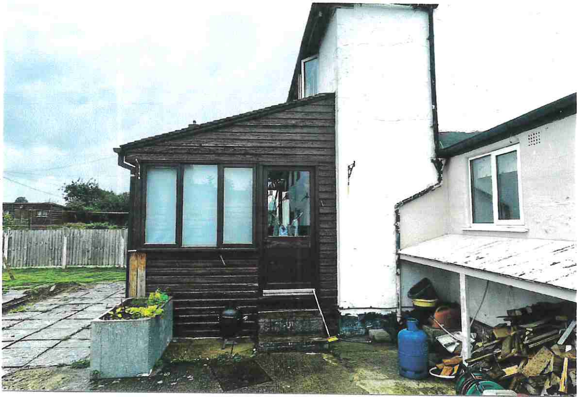
PHOTOGRAPH 6 - DETAIL OF THE EXISTING TIMBER CLAD CONSERVATORY WHICH IS TO BE REPLACED.
