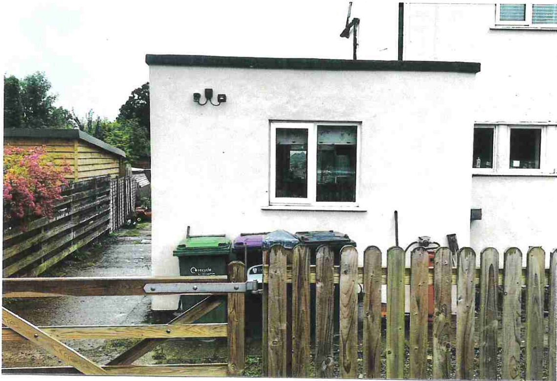
PHOTOGRAPH 2 - DETAIL OF THE EXISTING SINGLE STOREY FLAT ROOF UTILITY RANGE LOCATED AT THE SIDE OF THE PROPERTY.
