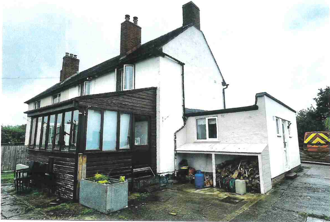
PHOTOGRAPH 4 - GENERAL VIEW FROM THE REAR OF THE PROPERTY WHICH SHOWS THE FLAT ROOFED SIDE RANGE AS WELL AS THE EXISTING CONSERVATORY.
