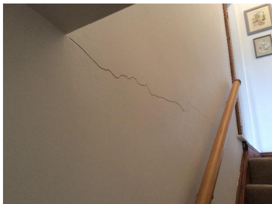
Picture 1: Rear extension/ house cracking
