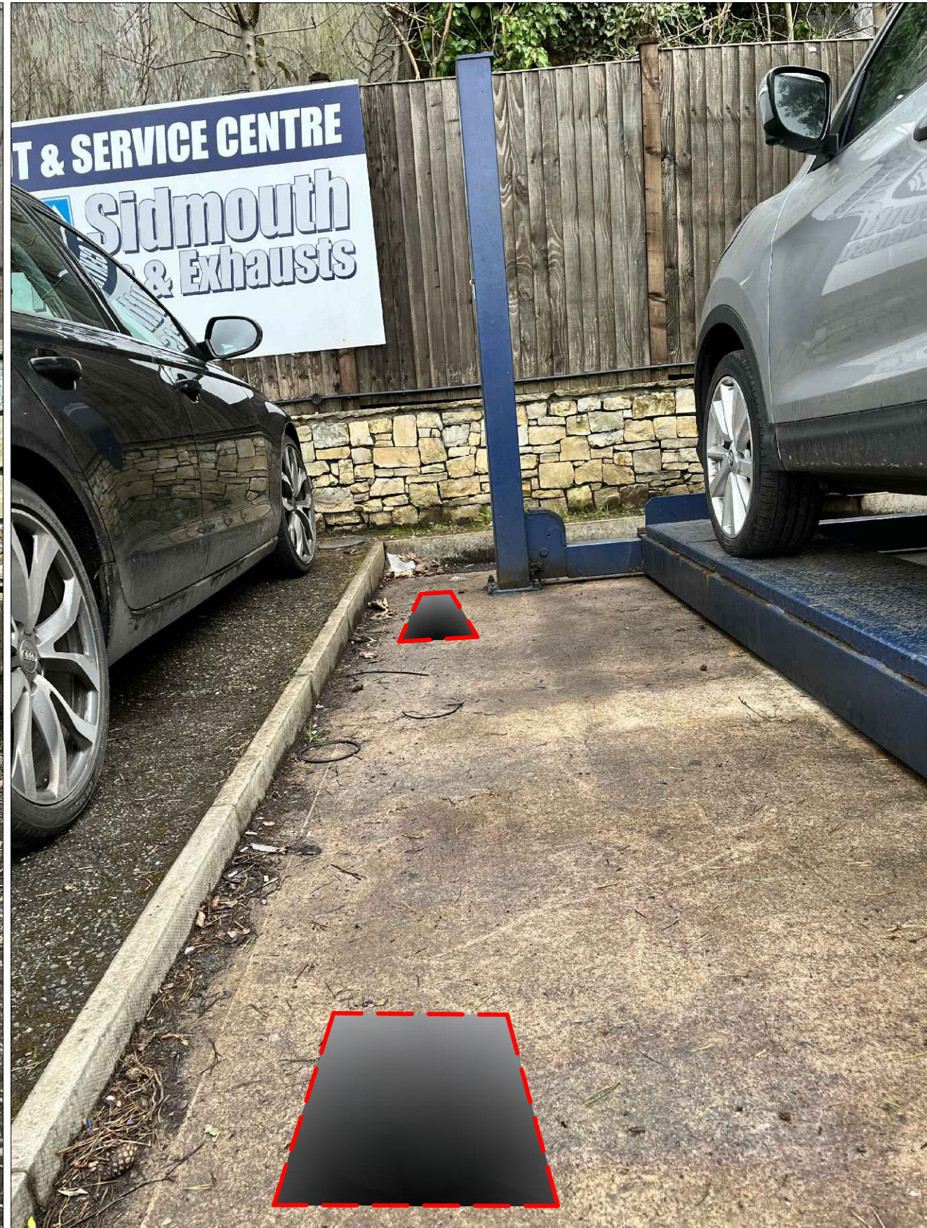
Photograph 2: Secondary hard surfaced area, hosting external ramp with very low likelihood of any rooting from Scots Pine T1 beneath. New pillars to be installed within this locatio, identified indicatively with red squares. Beams to be installed are 250 x 140mm I beams, as per adjacent existing building structure.
