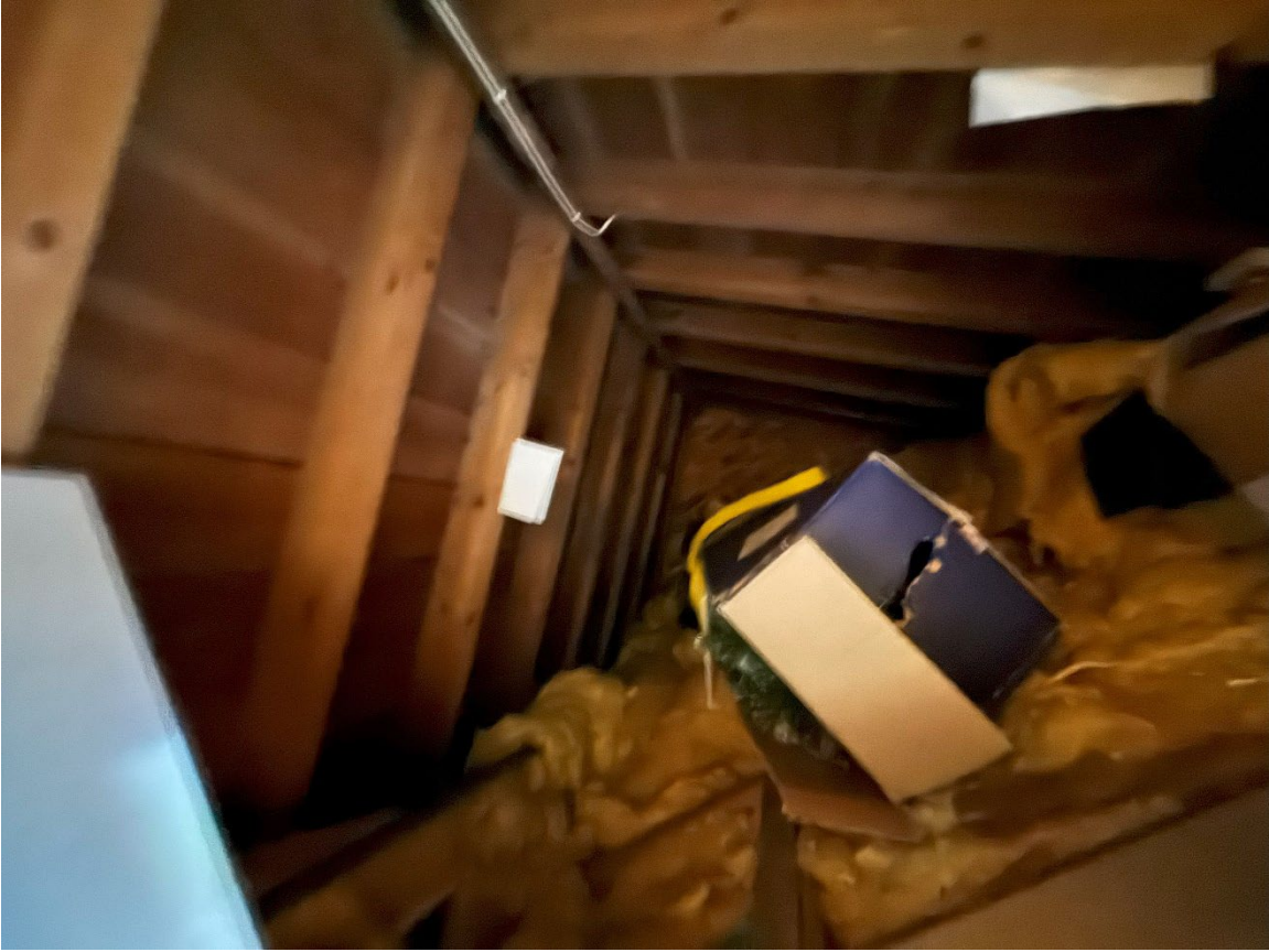
Figure 1 Existing Loft space
