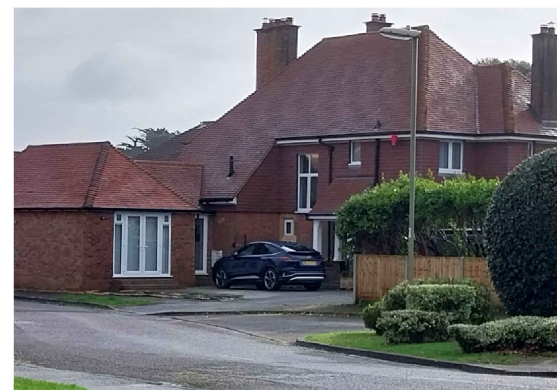
EXISTING IMAGE FRONT OF HOUSE
