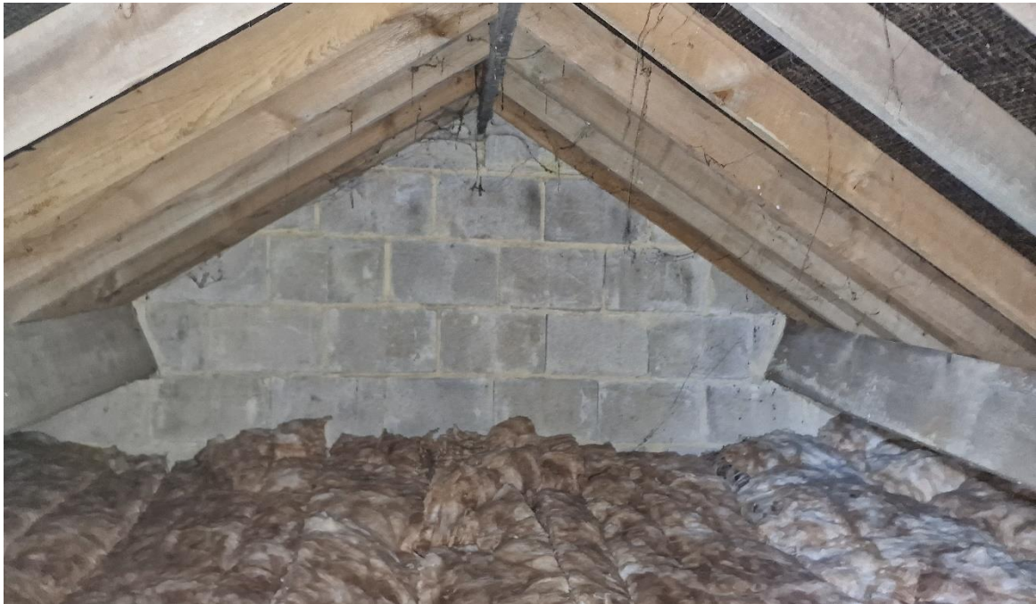
Picture 4: Showing the internal roof structure of the main house.
