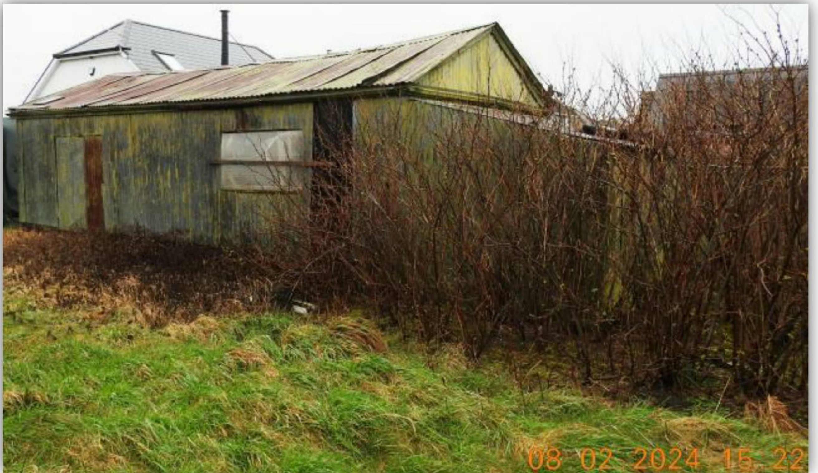
Dilapidated corrugated iron shed.
