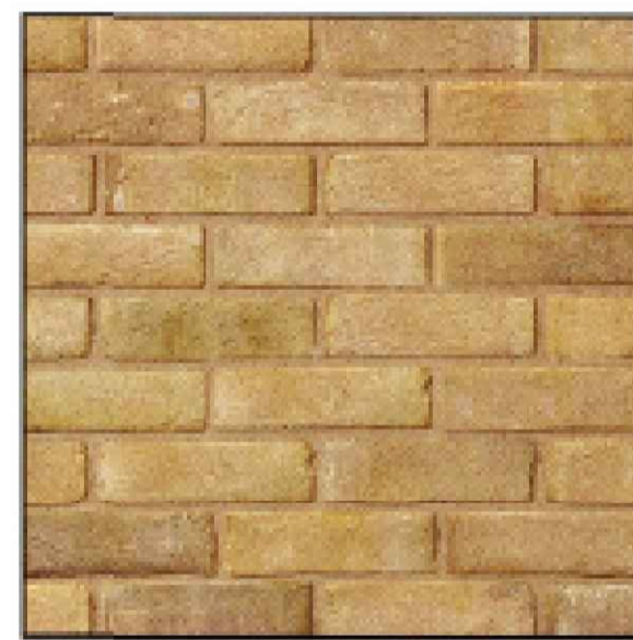
BRICKWORK Buff brick
