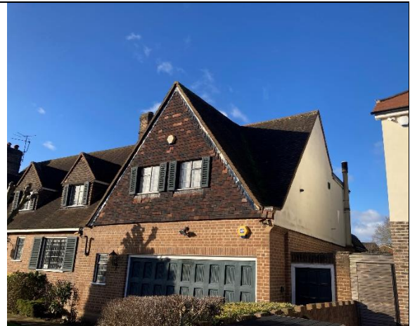
Photograph 2: North eastern view of building
