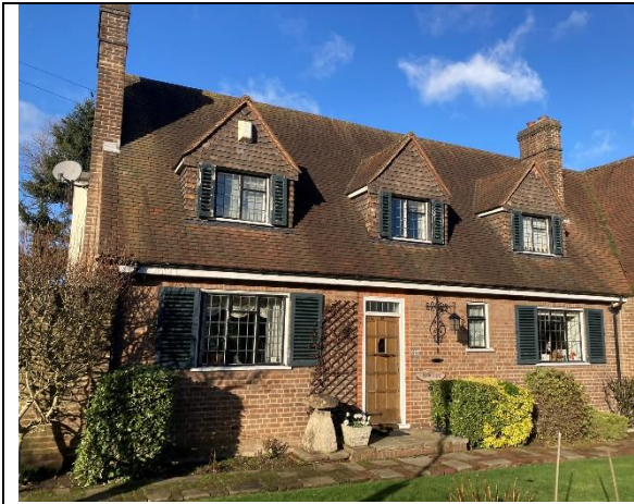
Photograph 1: Southeast corner of building.
