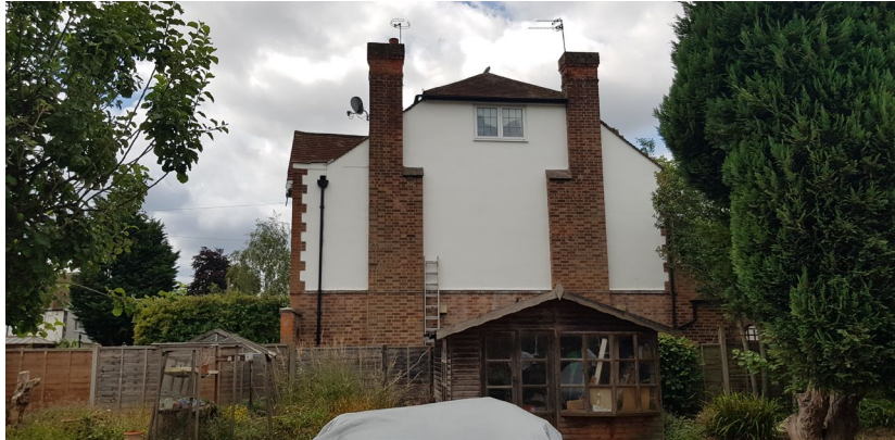
Figure 3. Window at 4 Spring Court Road facing proposed development
