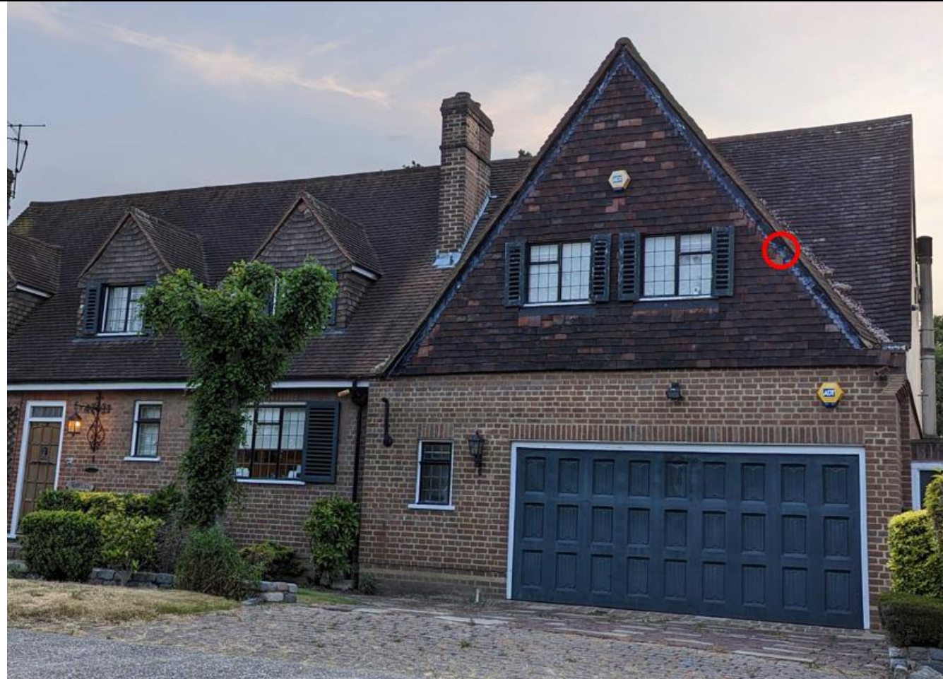
Figure 4. Emergence point (circled in red) of 1no. common pipistrelle at 21:47.
