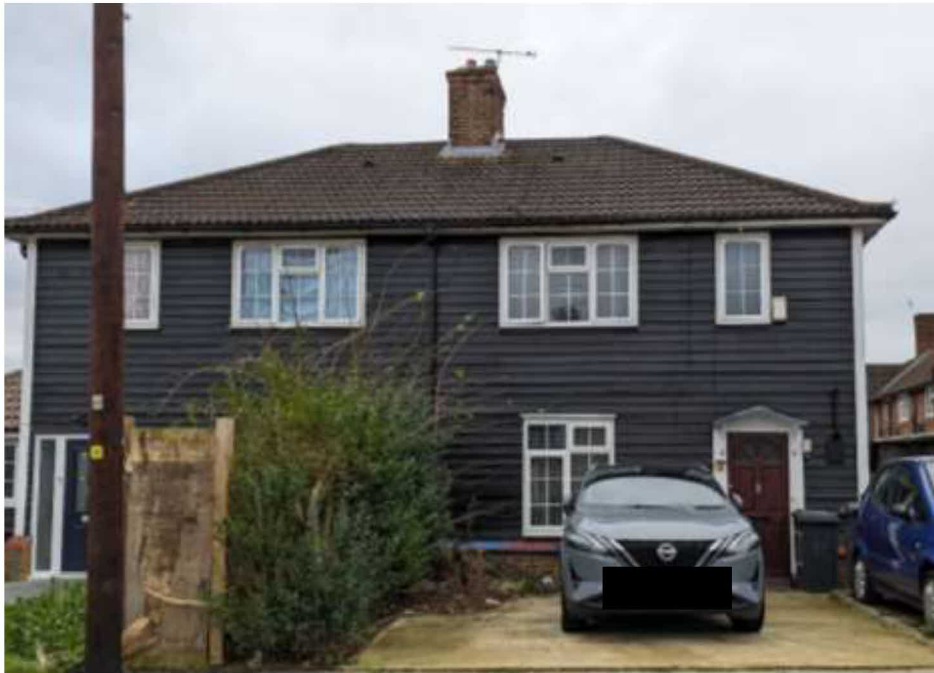
Fig. 15: Existing windows are uPVC with internal glazing bars and ‘chunky’ openers which do not enhance the properties. The ground floor windows to each house do not match in fenestration design.
