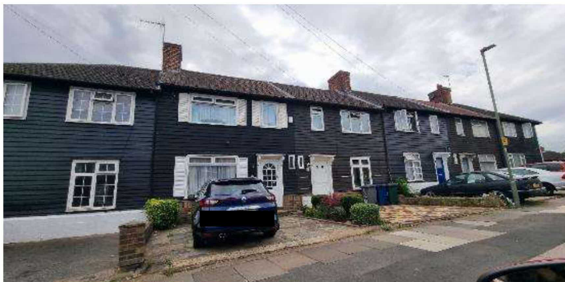
Fig.3: An example of a terrace of timber construction houses, with feather edge boards applied over a timber frame
