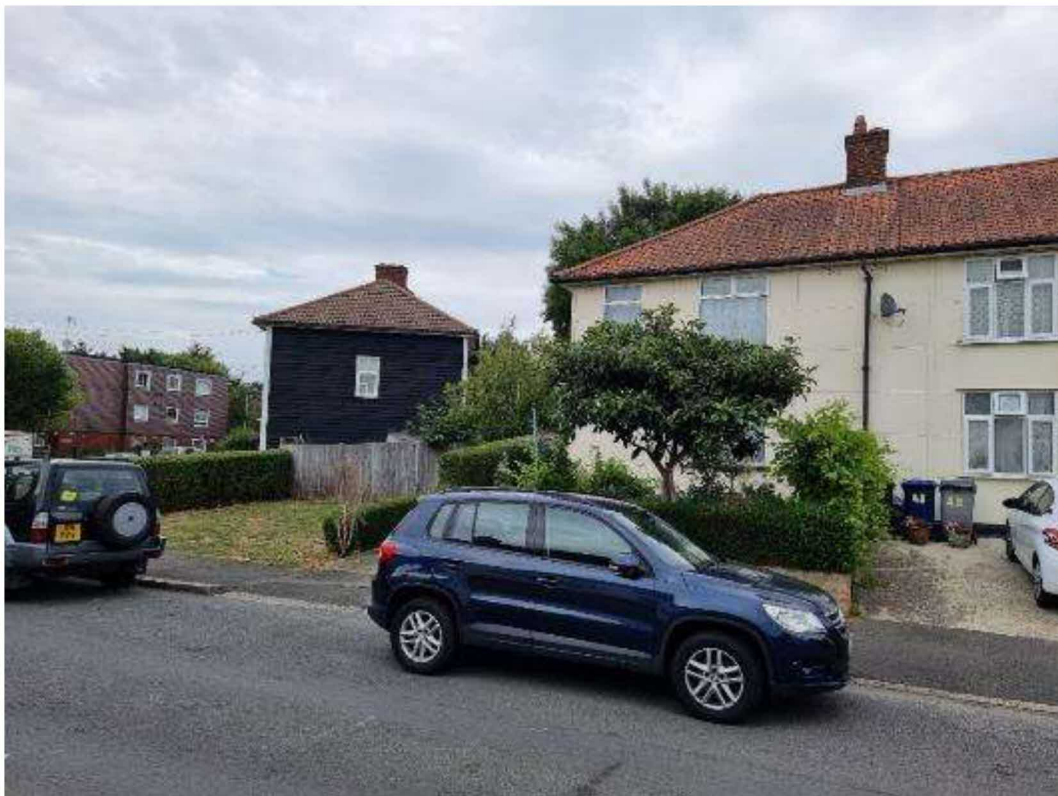
Fig.5: Timber properties and steel properties positioned next to each other on a corner with grass verges, a typical layout style for the area.
