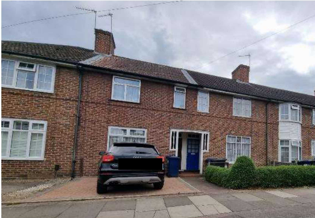
Fig.4: An example of more conventional brick construction properties.
