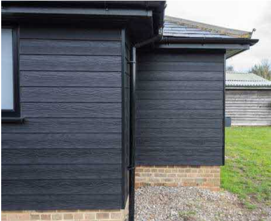
Fig.13: Proposed Cedral Lap cladding in woodgrain to match existing boards
