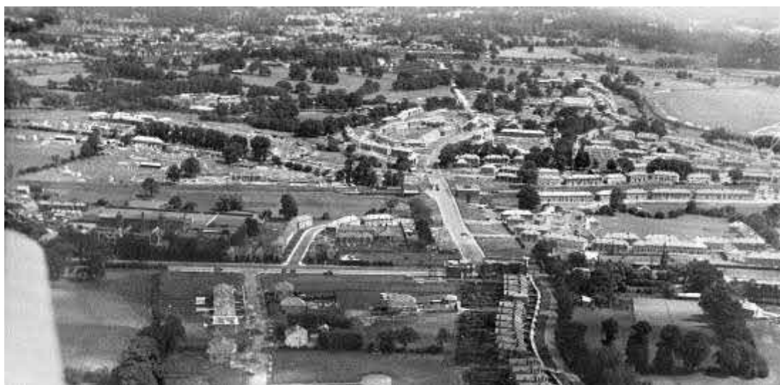
Fig.8: The Watling Estate under construction in 1927. Source: Britain from Above.
