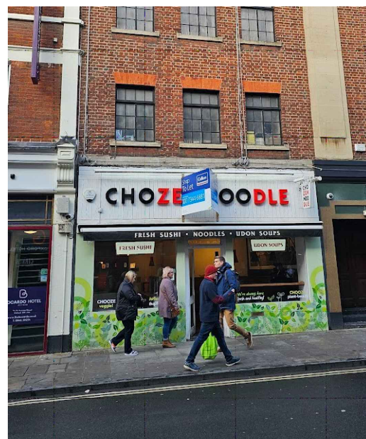
Existing shop front photo
