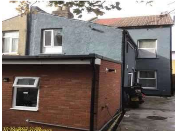
Photo of Rear Elevation
