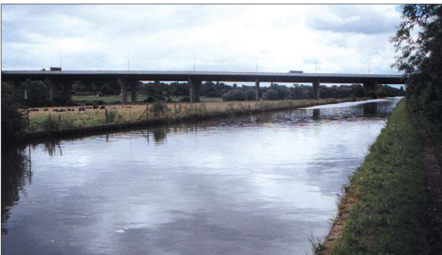
• Grand Union Canal and M25 viaduct (J. Billingsley)
