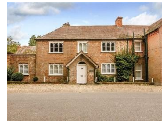
Fig 2: 1 The Grange - West Elevation Street View
