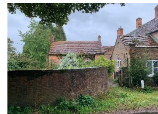
Fig 3: 2 The Grange - West Elevation Street View
