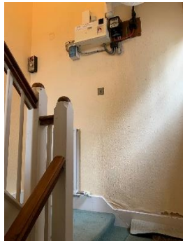
Fig 32: Upper Ground Floor Staircase
