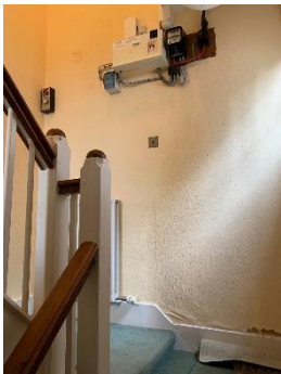
Fig 9: Upper Ground Floor Staircase
