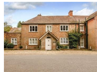
Fig 2: 1 The Grange - West Elevation Street View
