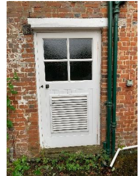
Fig 12: Upper Ground Floor External door to Plant Room
