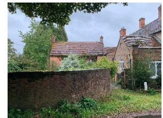
Fig 3: 2 The Grange - West Elevation Street View
