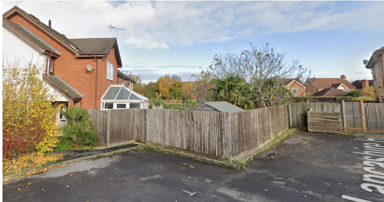
View of the fence for No.6 along the southern boundary/car park.
