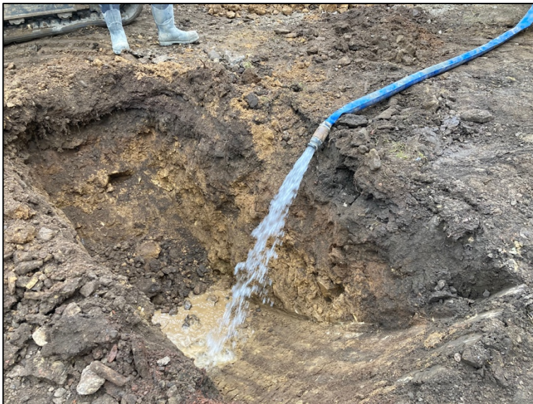
View of TP1 pit
