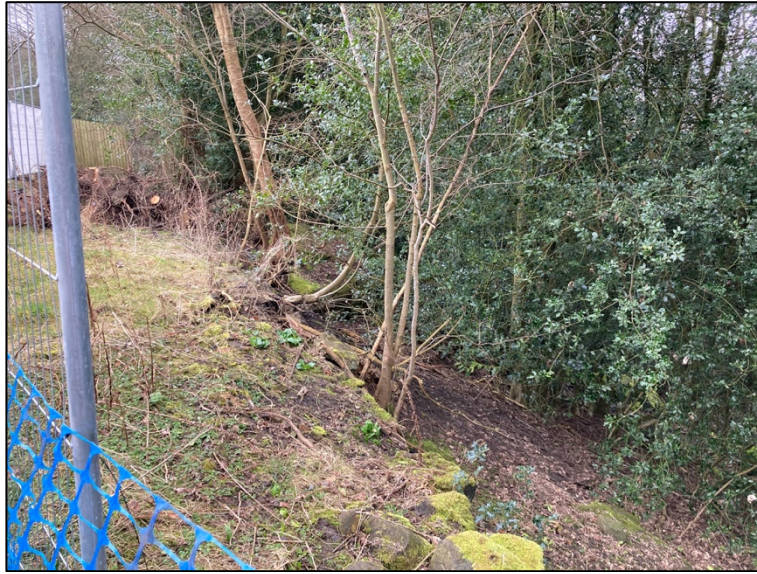
View of southern boundary showing slope condition
