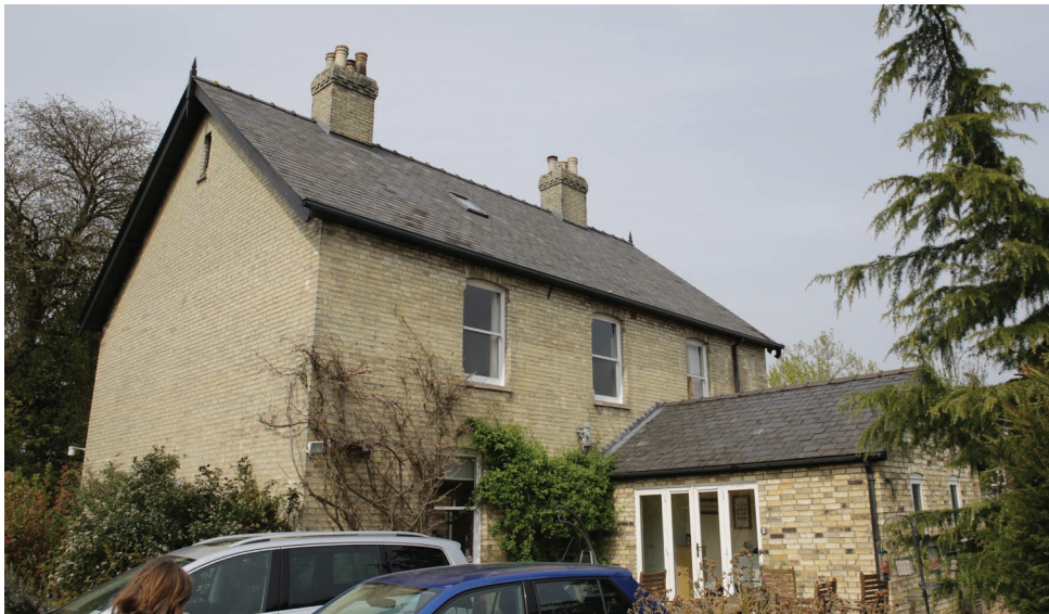
Fig 12. Location of new extension proposal at the rear of No. 27 High Street
