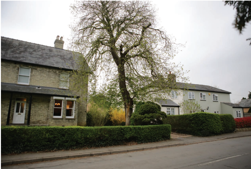
Fig 5: Relationship between No. 27 High Street and No. 29 High Street.
