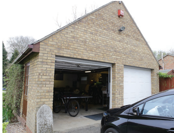
Fig 11. Existing garage of No. 27 High Street
