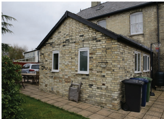
Fig 8. Previous rear extension to No. 27 High Street
