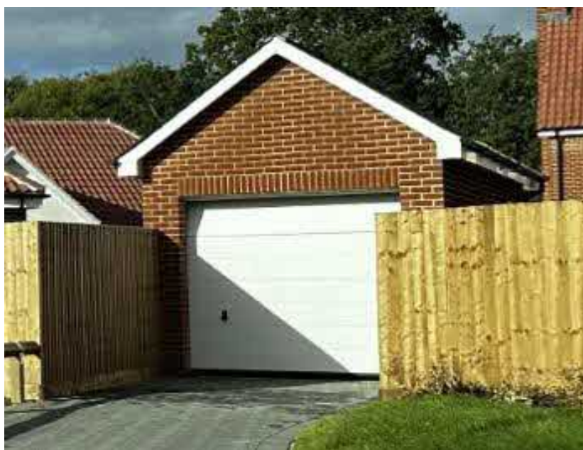
Photo showing an existing garage which lies on the boundary with 1 The Wickets.
