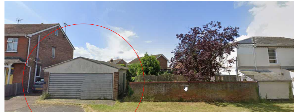
existing view looking south across spring road
