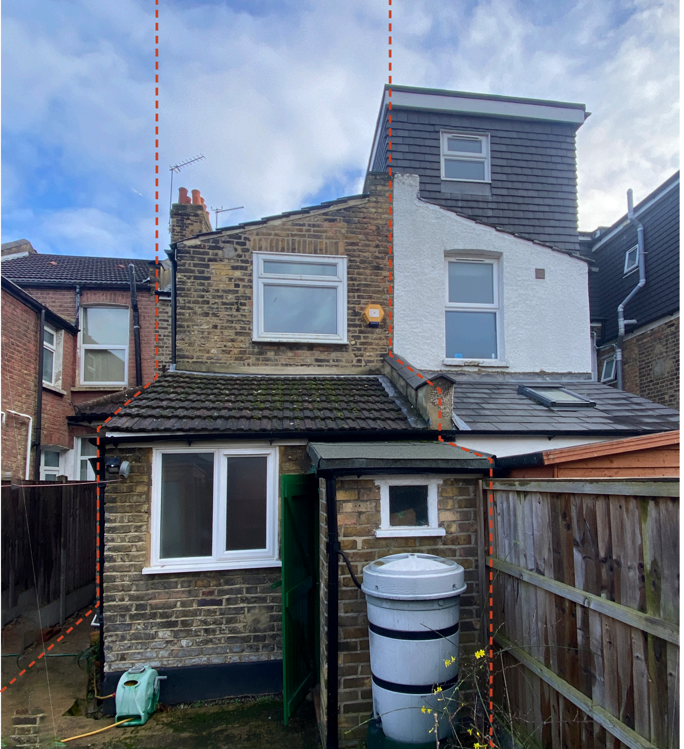
Rear elevation showing the boundary, edge conditions and neighbouring properties.
