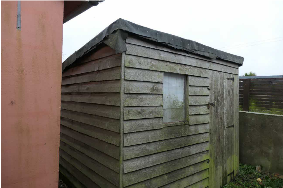
Photo 13, north and east aspects of building three, looking southwest.
