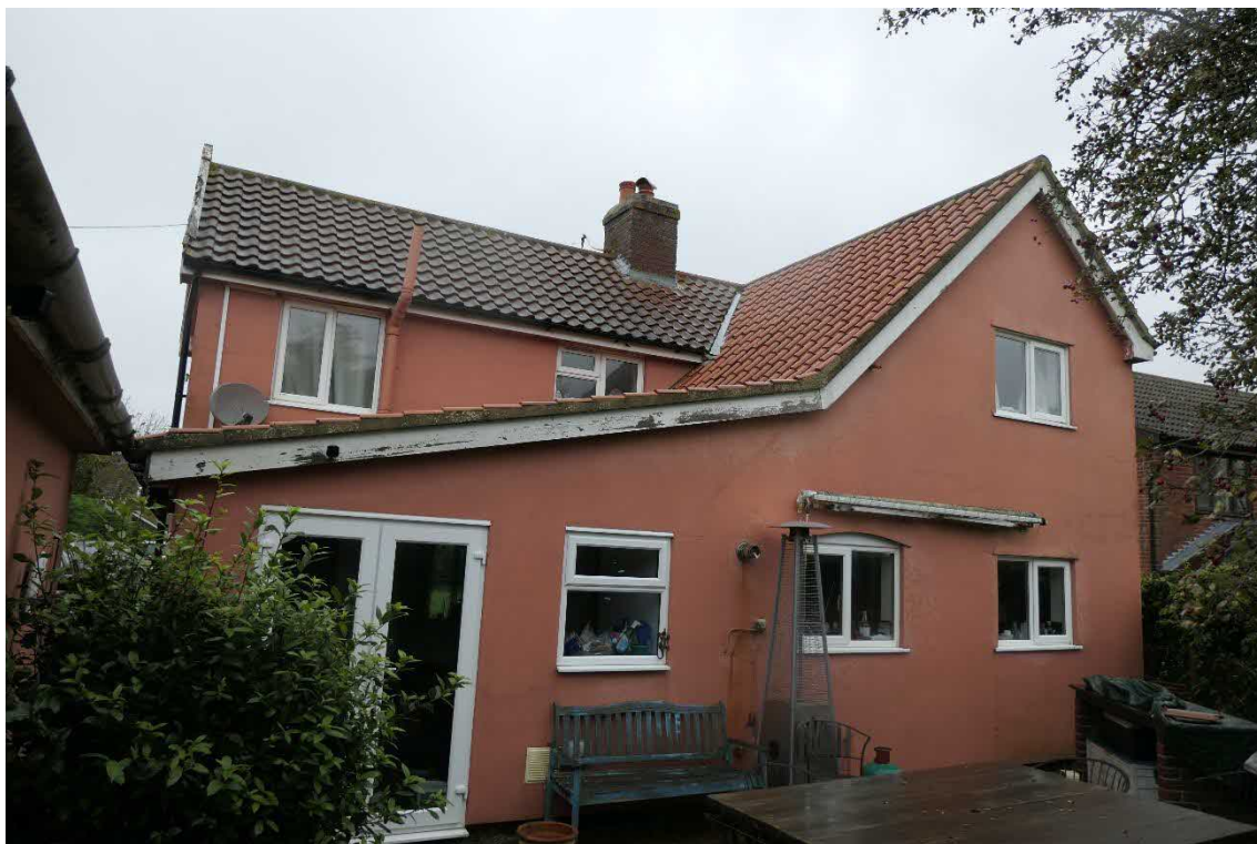
Photo 8, south aspect of building one, looking north.
