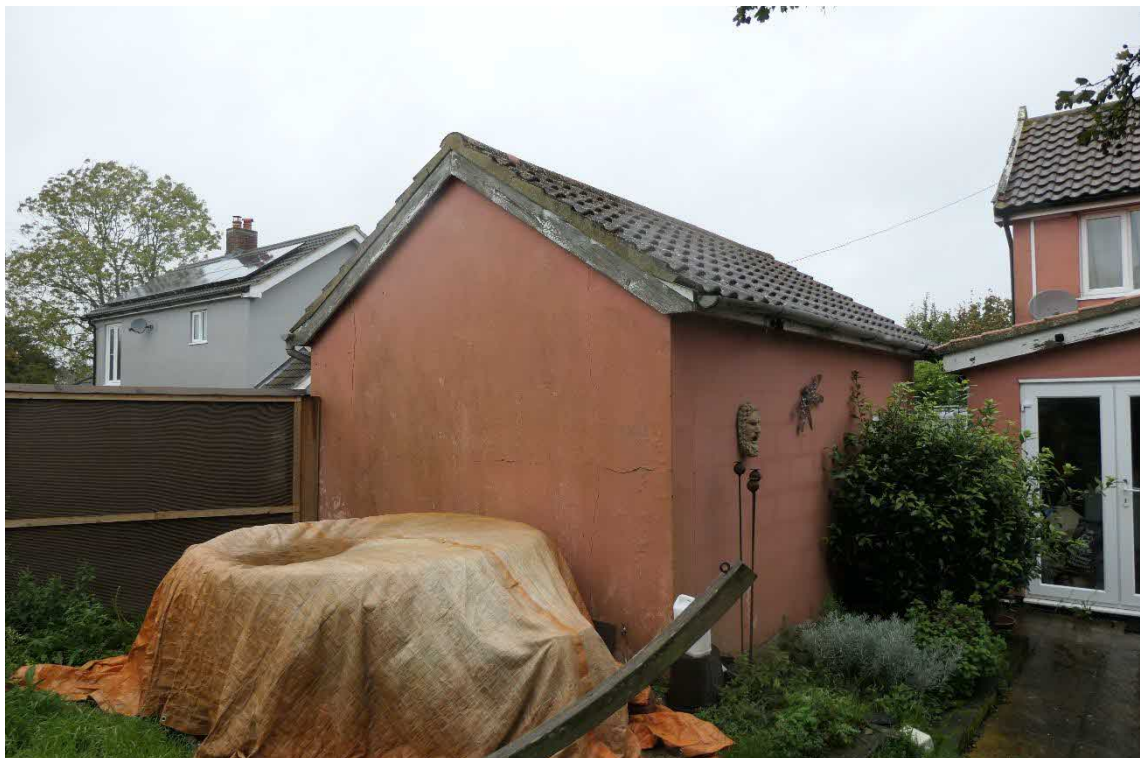
Photo 12, south and east aspects of building two, looking northwest.
