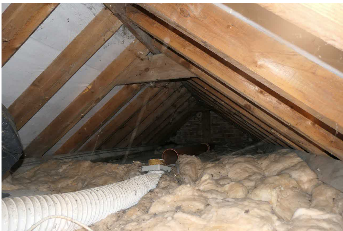
Photo 9, internal view of building one, looking west.
