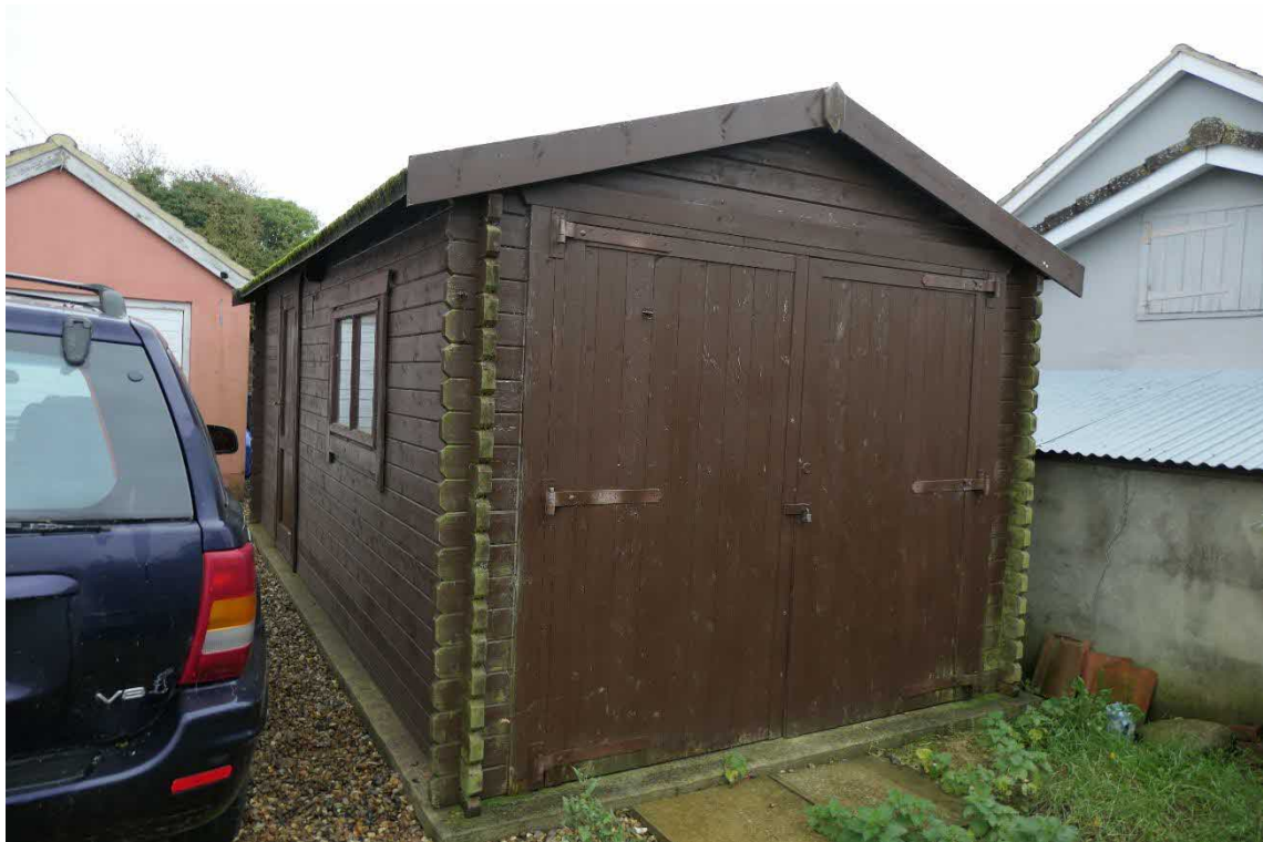
Photo 14, north and east aspects of building four, looking southwest.
