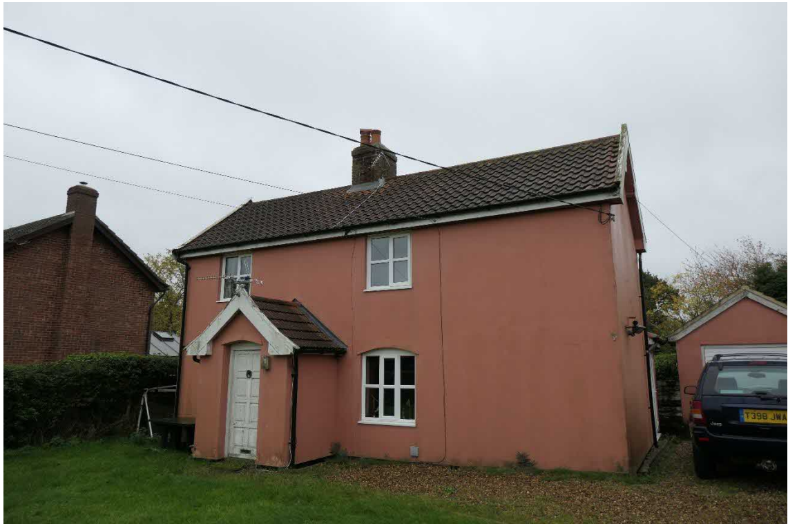
Photo 7, north and west aspects of building one, looking southeast.
