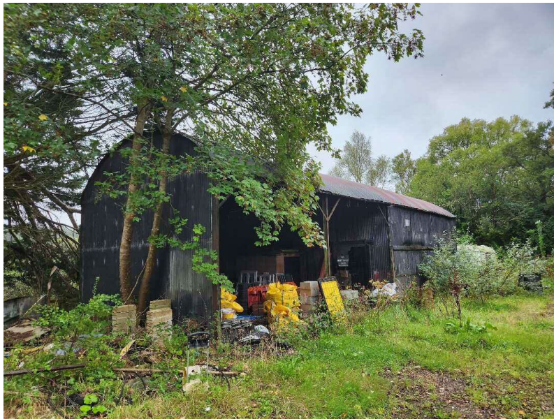
Figure 2: Photograph of existing building.
