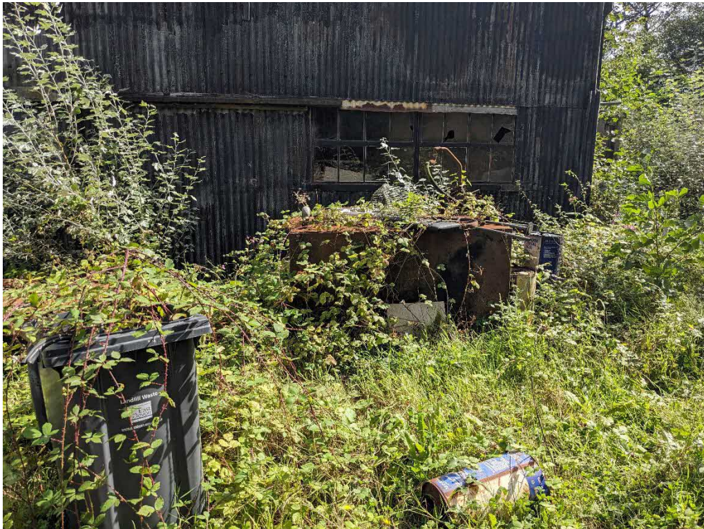
Photograph 5: View of old oil drums adjacent to building.
