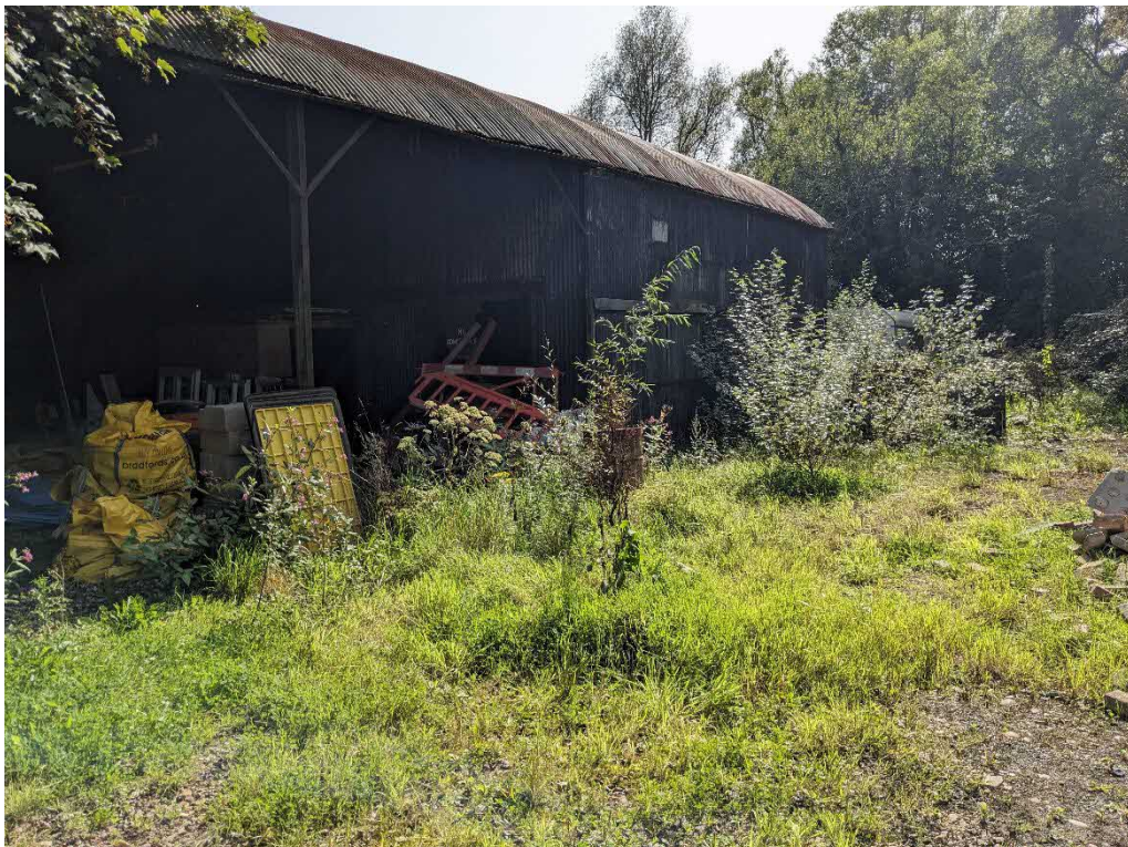
Photograph 2: View of the building looking south-west.
