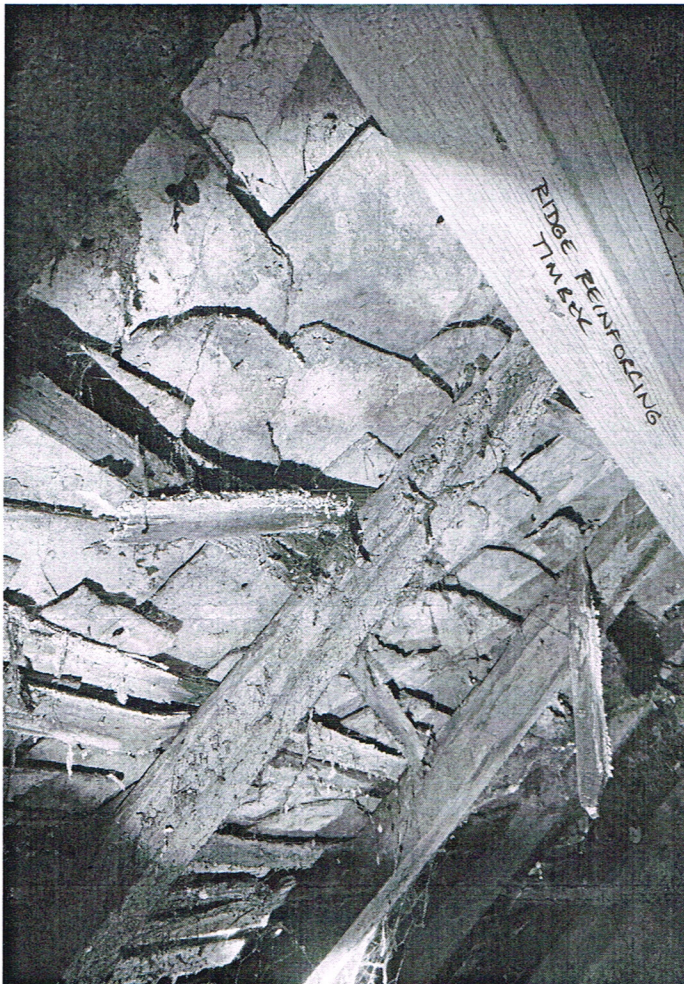
NORTHERN REAR SLOPE - SHOWING MORE DECAY OF TIMBERS AND SLATE
