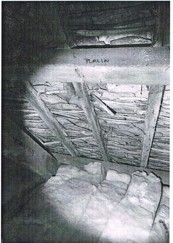
NORTHERN REAR SLOPE - SHOWING DECAY OF TIMBERS AND SLATE ABOVE CEILING.
