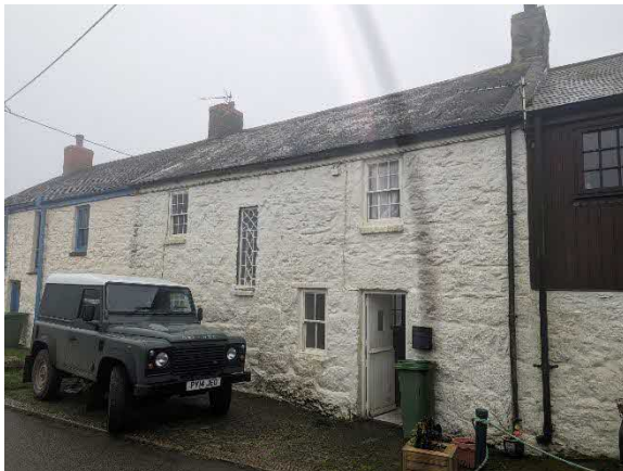
Photo 1. Showing the cottage from the north
