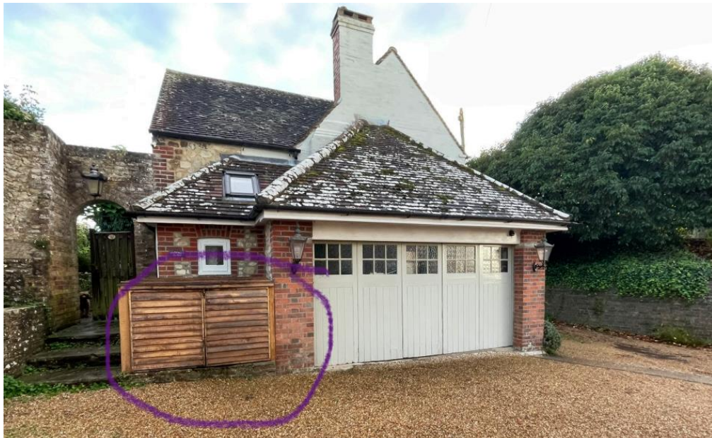
Fig.7 photo of the existing side north elevation
