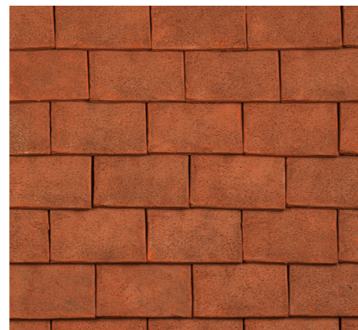
Left and fare left: samples of handmade peg tiles will be sought to match the existing tiles.
