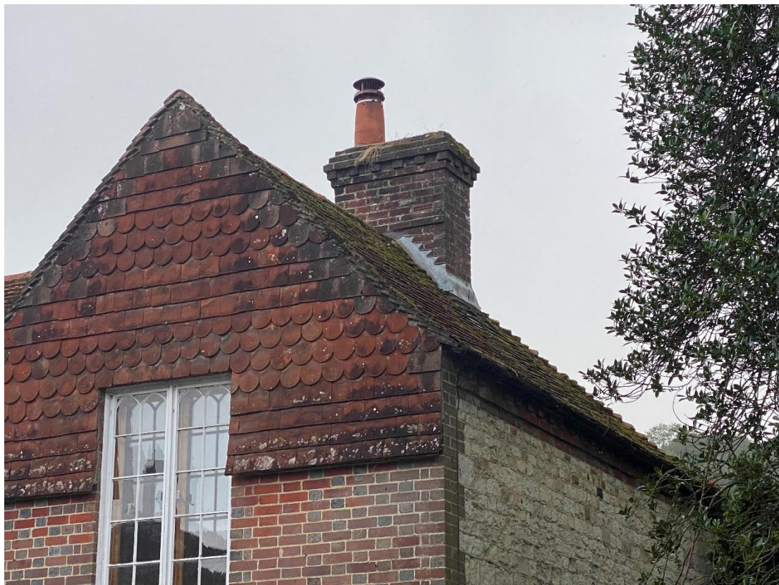
Figure 2. Eastern and northern elevations looking west.
