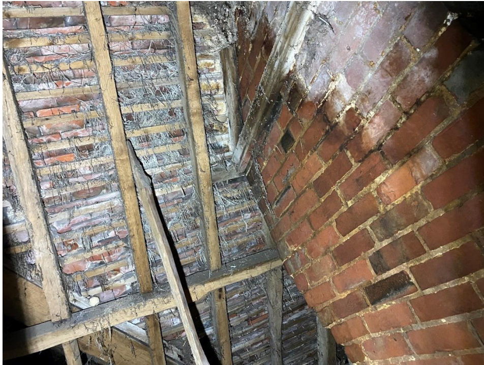
Figure 7. West face of main chimney looking east.
