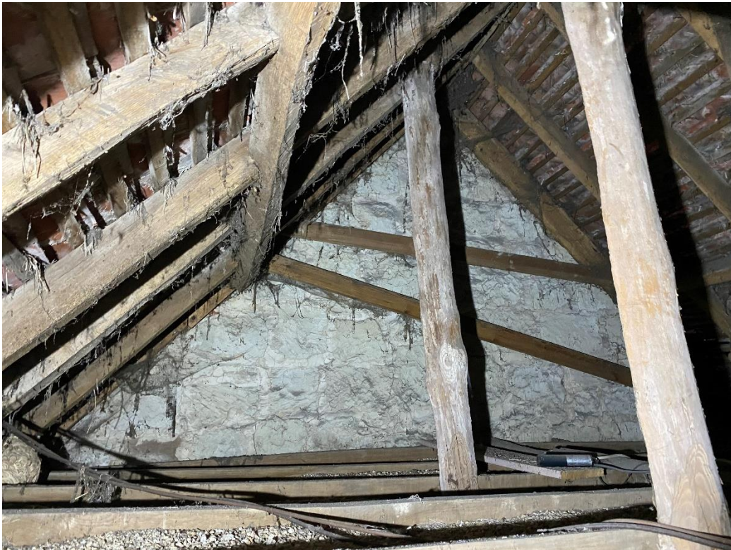
Figure 6. Looking south of south wall of loft
