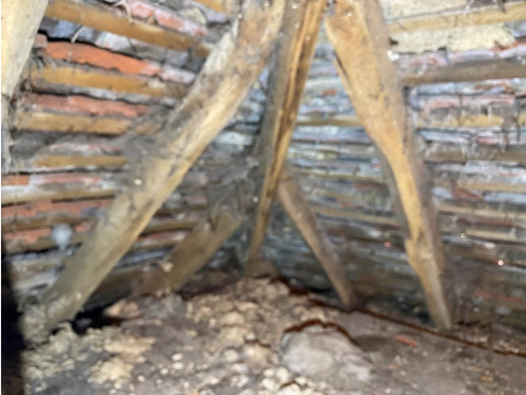
Figure 5. Looking north at north corner roof.
