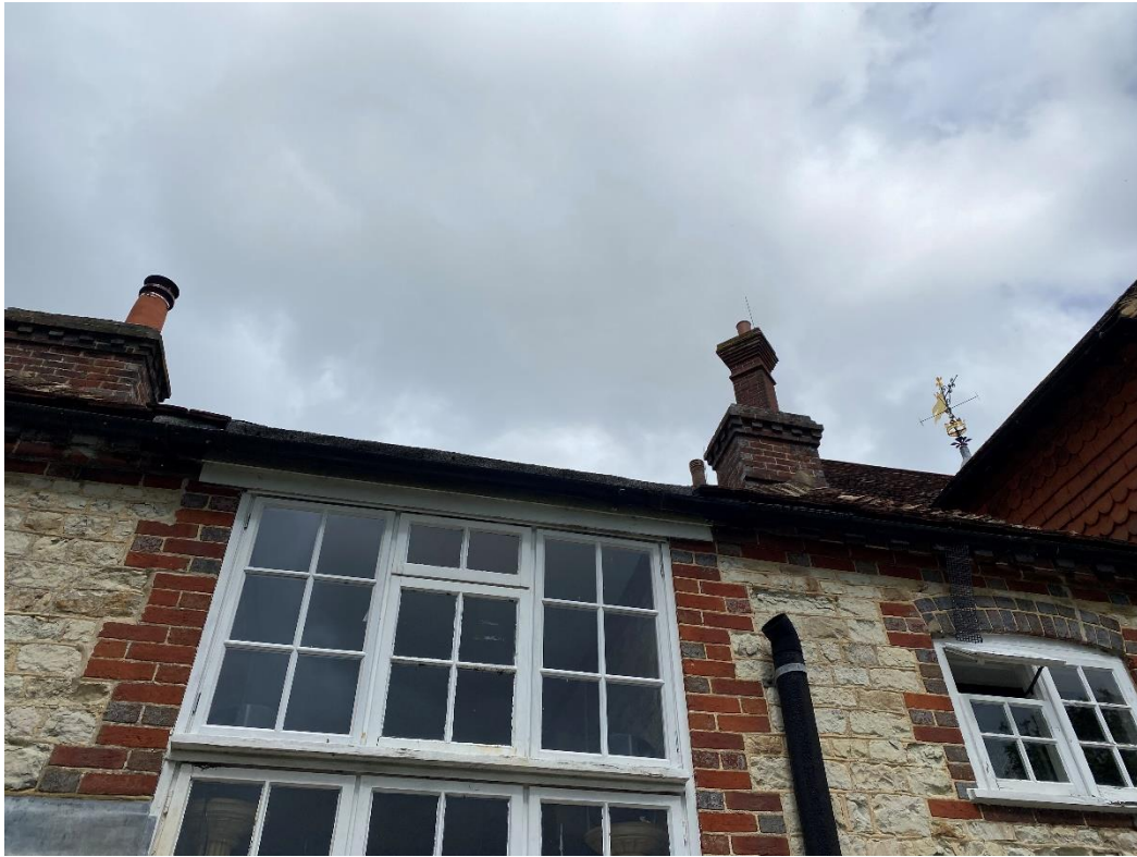
Figure 3. Western elevation looking southeast.
