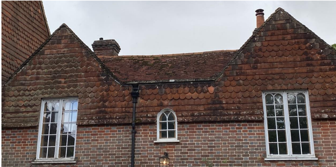
Figure 1. Eastern elevation looking west.
