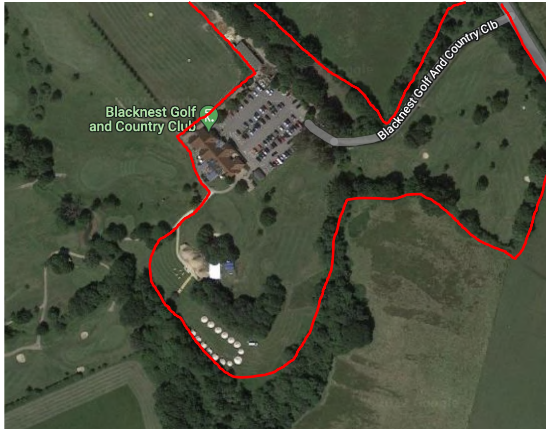
Figure 1: Aerial map showing areas of proposals, showing tipis erected and a previous event using temporary camping 'tipis' for additional overnight accommodation —copyright Google Maps 2022
