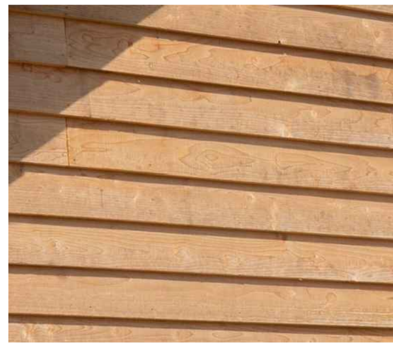
Above. Natural Douglas fir cladding to carport.
