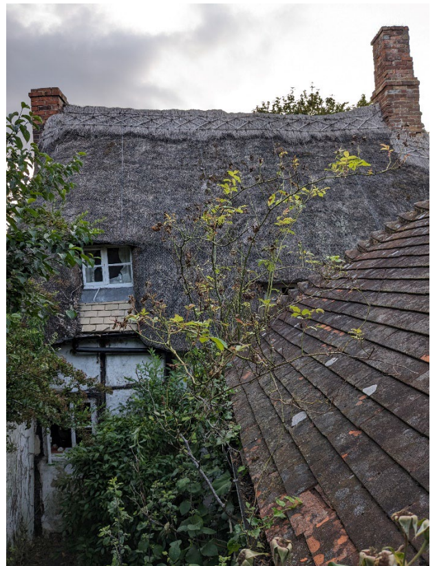
Photo 3 – Rear view of Chimney
