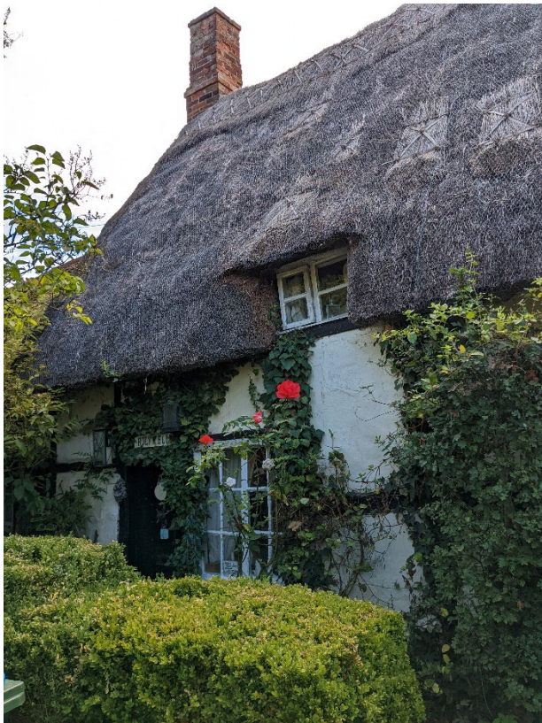
Photo 2 – Front view of Chimney
