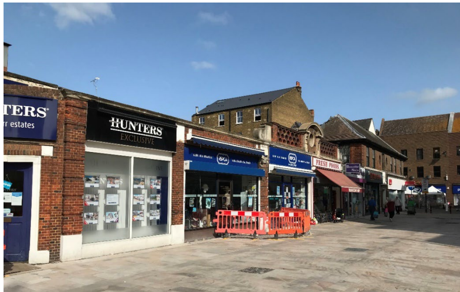
Photo 2: Nos. 1-5 Market Place
