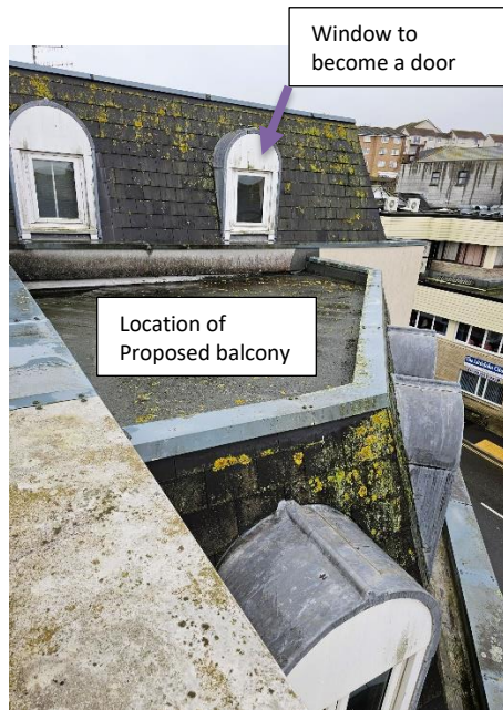
Fig 1 – existing flat roof (flat 9)
