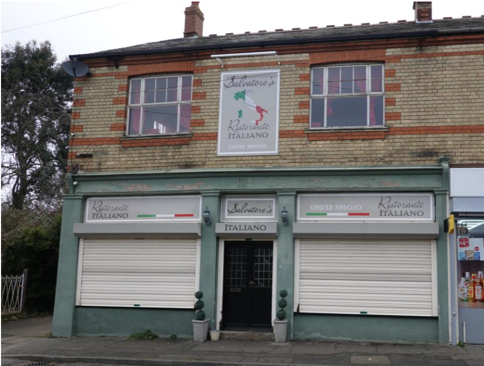
Figure 5. Adjacent property – note the roller shutters.
