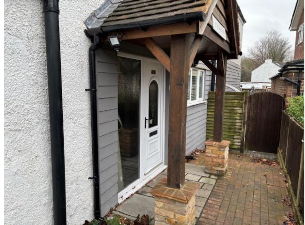
Fig 6. Image showing the front door of the site.
